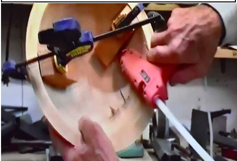
Clamps hold the contoured blocks in place while hot glue is applied.
